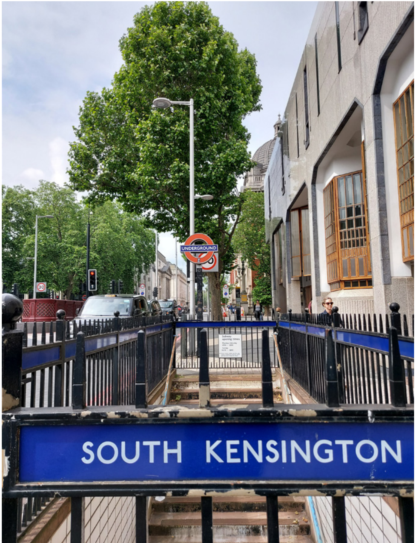
FIGURE 5 SOUTH KENSINGTON STATION. CREDIT: EXHIBITION ROAD CULTURAL GROUP
