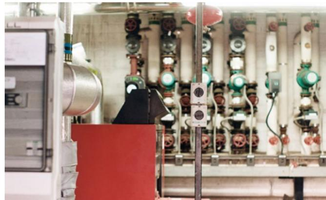
Above: Inside the boiler room at County Hall, where a heat exchanger unit has replaced a gas boiler
